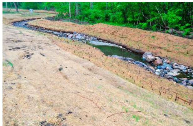
Figure 4. Area with live stakes along County Farm Drain, Spring 2012. Photo by Dan Bruell, used with permission.
