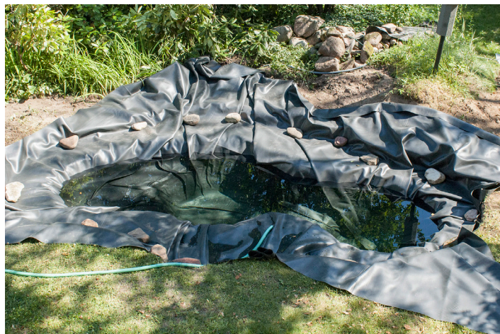
Figure 2. Pond liner in place and filling.
