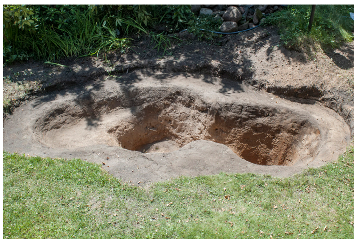
Figure 1. Holes for pond dug three feet deep.
